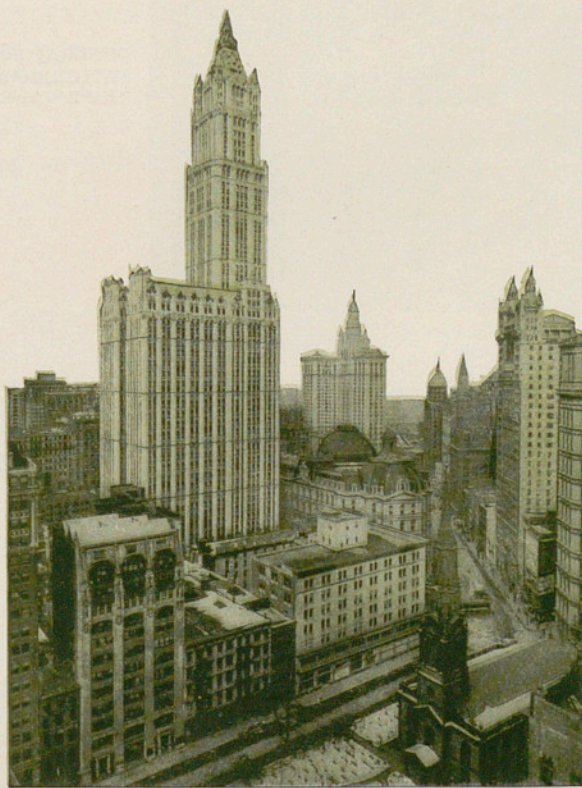
VIEW FROM THE SOUTHWEST
