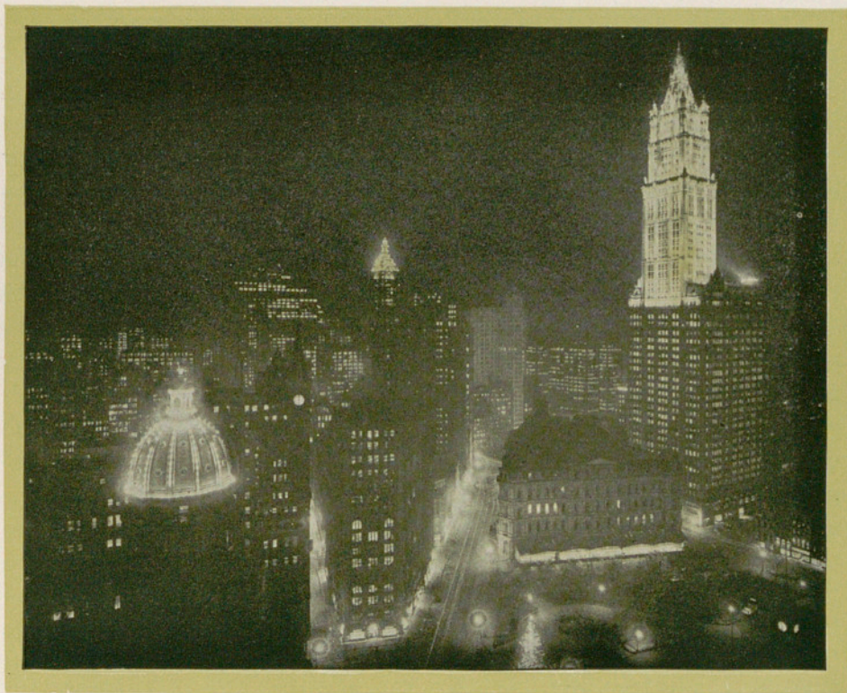
THREE TOWERS OF LOWER MANHATTAN AT NIGHT
