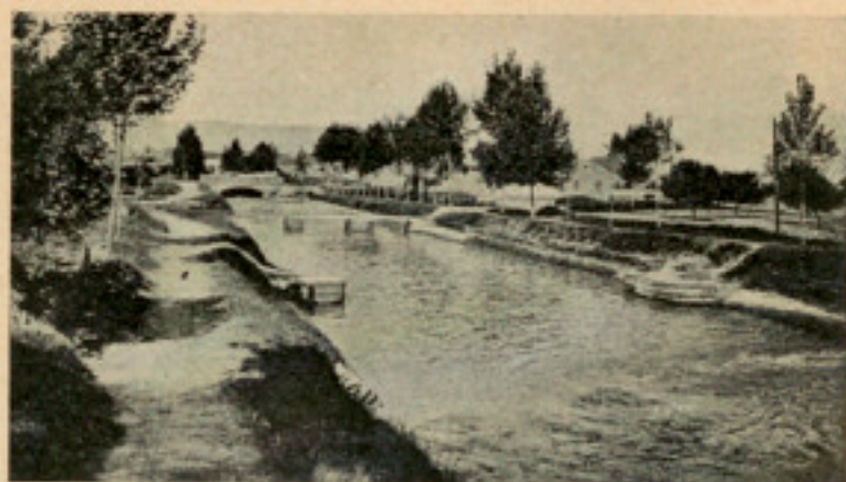
Fig. 6. — Cana principal de recs, Amposta
